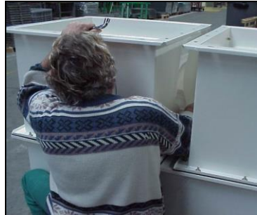
In between housings, flange access is easier from the back side, using a ratchet. Do not block bolts yet at this point.
