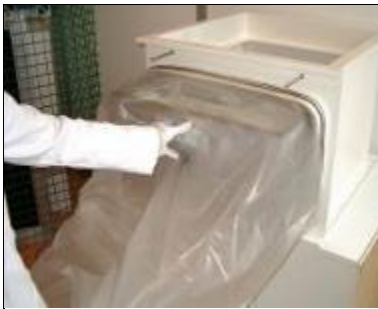
Push gently until hitting the stop. The lever shape ensures that only a fully inserted filter can be locked
