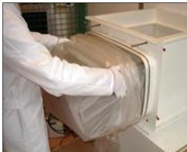
Extract the filter into the bottom of the bag
