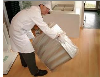
Turn the filter over and place in front of the housing
