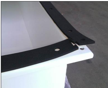
Place gaskets on the flange, aligning flange and gasket holes. Interlocking connectors (modular gaskets only) facilitate placement.
