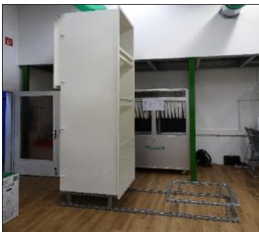
Place 1 st collector on the support stand.
