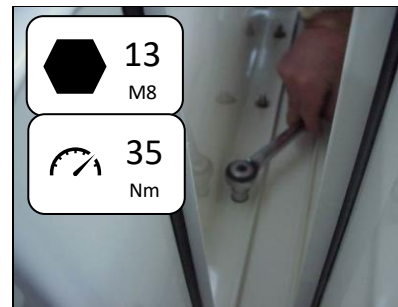
Tighten to 35 Nm torque.
