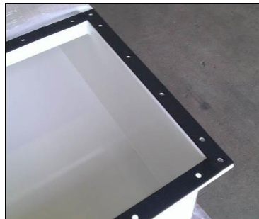
Place gaskets on the flange, aligning flange and gasket holes. Interlocking connectors (modular gaskets only) facilitate placement.
