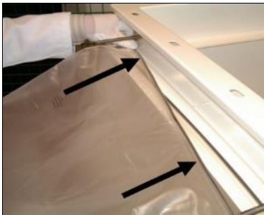
Slide the new bag over the stub and the collar
