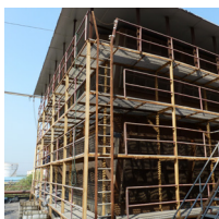
Pictures from the original filter house. Dismantling and erection of the new barrier type Inlet Air System
