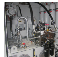
Retrofitted diverter damper system with replaced expansion joints, actuator and HPU.
