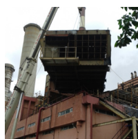
Pictures from the original filter house. Dismantling and erection of the new barrier type Inlet Air System
