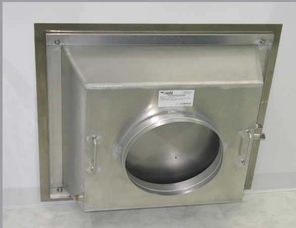
Top photo: Pharmaseal Exhaust Housing installed in a cleanroom wall offers an aesthetically pleasing room side appearance. Bottom photo: Same unit with testing shroud mounted on the Pharmaseal frame for overall filter efficiency testing from within the room.
