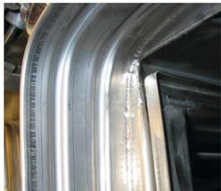
Each filter access port includes a ribbed bagging ring assembly for attachment of an 8-mil changing bag of polyvinyl chloride (PVC) construction. The bagging ring is continuously welded and hemmed to prevent damage to the bag.
