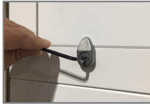
2 - Loosen Panel Stops with 4mm Hex Key
