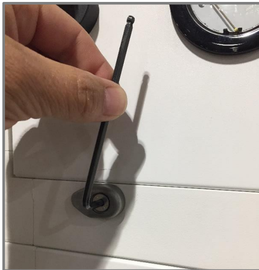
3 - Rotate Panel Stops to Open Position
