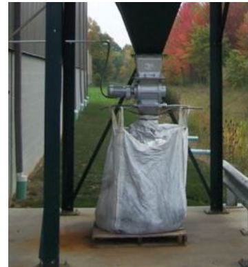
Discharge adapted to the quantity and type of dust collected
