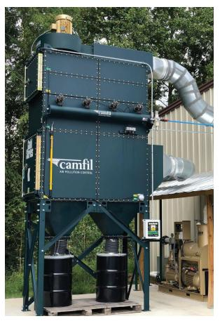
Eight-cartridge dust collector captures laser cutting fumes from an automated tube cutting application.
