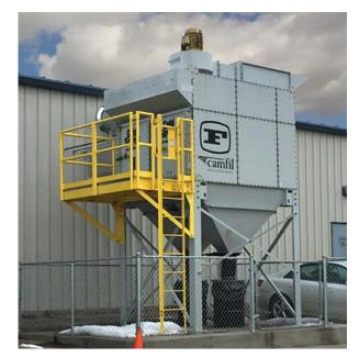
A Farr Gold Series® 20-cartridge collector captures fumes from three automated flat laser cutting machines.
