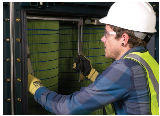
Gold Cone X-Flo filter cartridges are quickly and safely changed out.
