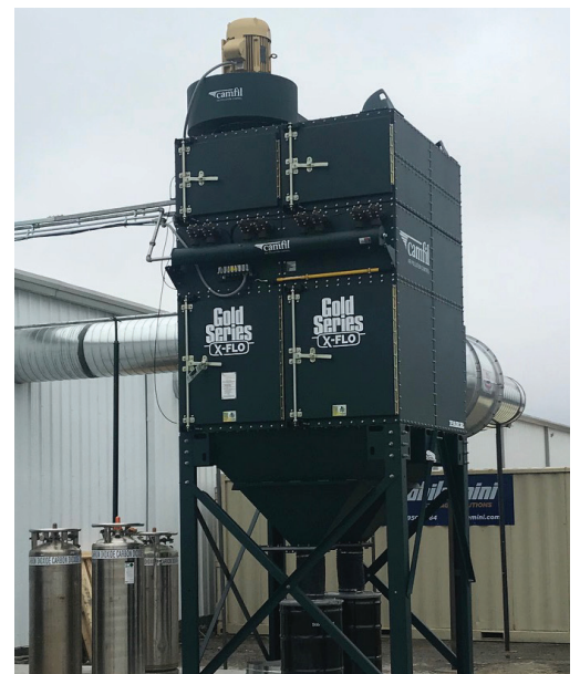
This Gold Series X-Flo dust collector is used to safely capture welding fumes at their source. An integrated safety monitoring filter is installed so that air can be recirculated back into the building.
