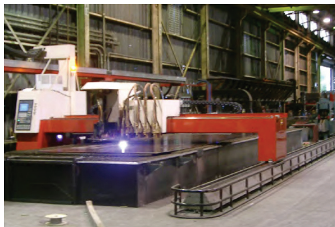
Top photo shows poor air quality during a dry plasma cutting operation, before filtration has been applied. Bottom photo shows the same shop after a high efficiency dust collector has been activated to capture smoke and fumes.
