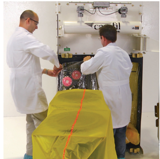
Bag-in/bag-out (BIBO) filter change is performed as part of a surrogate test. Surrogate testing helps predict real-world performance of dust collection equipment in containment applications.
