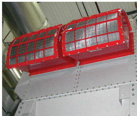
Explosion vents and flameless venting are two types of explosion protection system that mitigate combustible dust explosions in dust collectors.
