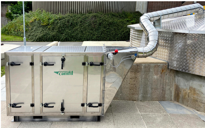
HDC unit with pre-filters and fan that cleans the air at the concentration tank
