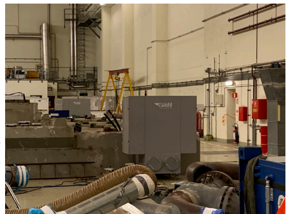
Air Cleaner CC 6000 in use at the plant
