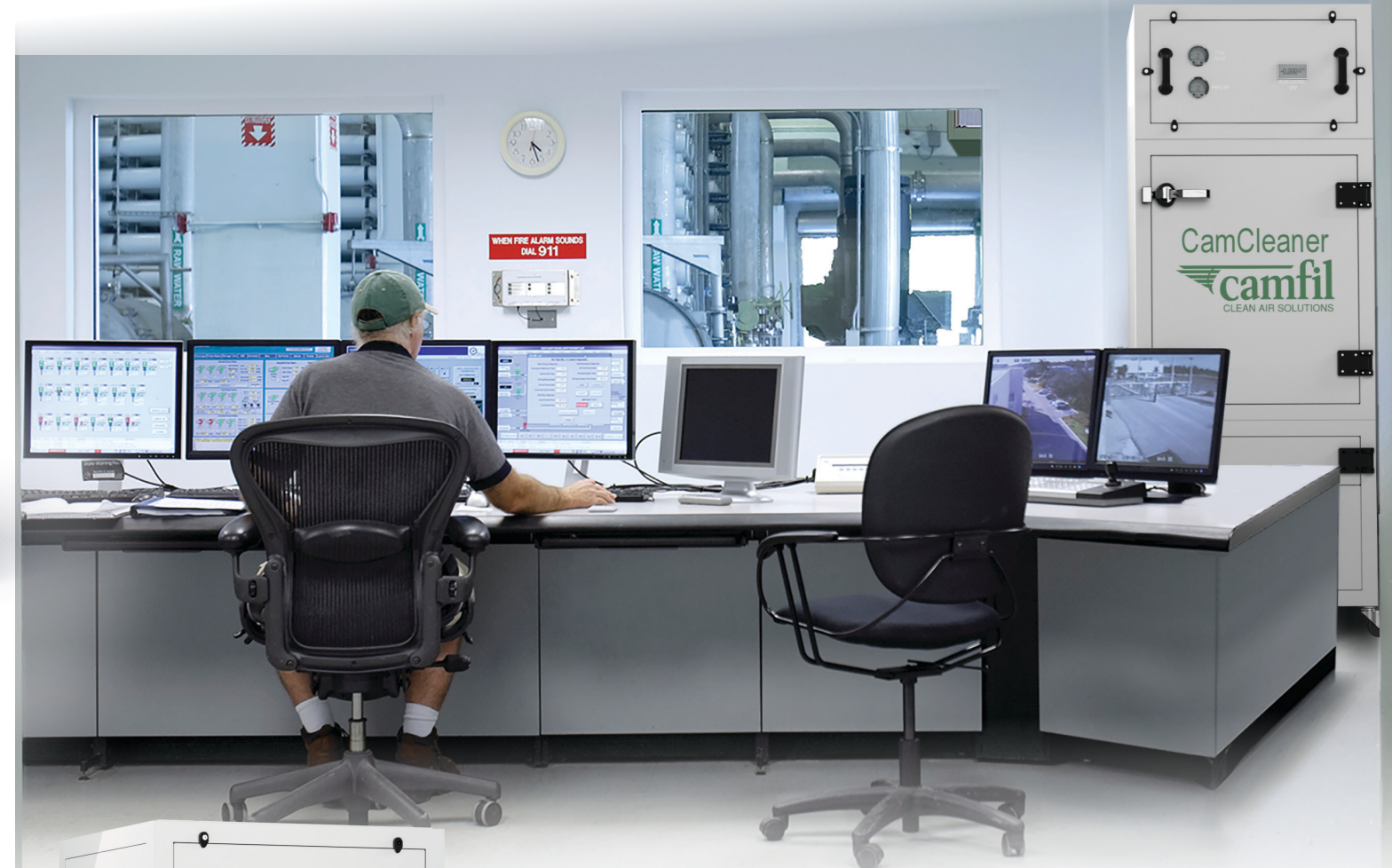
CamCleaner Vertical with molecular filters in a control room.
