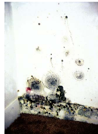
Water and nutrients offer a fertile breeding ground for mold. Flood damage should be repaired or replaced as soon as possible to prevent cross-contamination.
