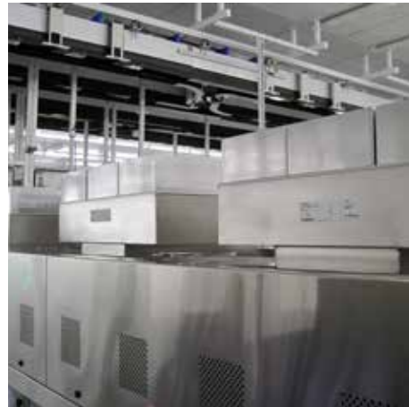
AMC filtration on top of process equipments
