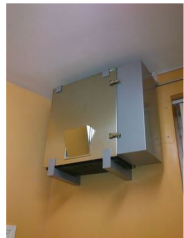
MIXED INTAKE RECIRC AND OUTSIDE
